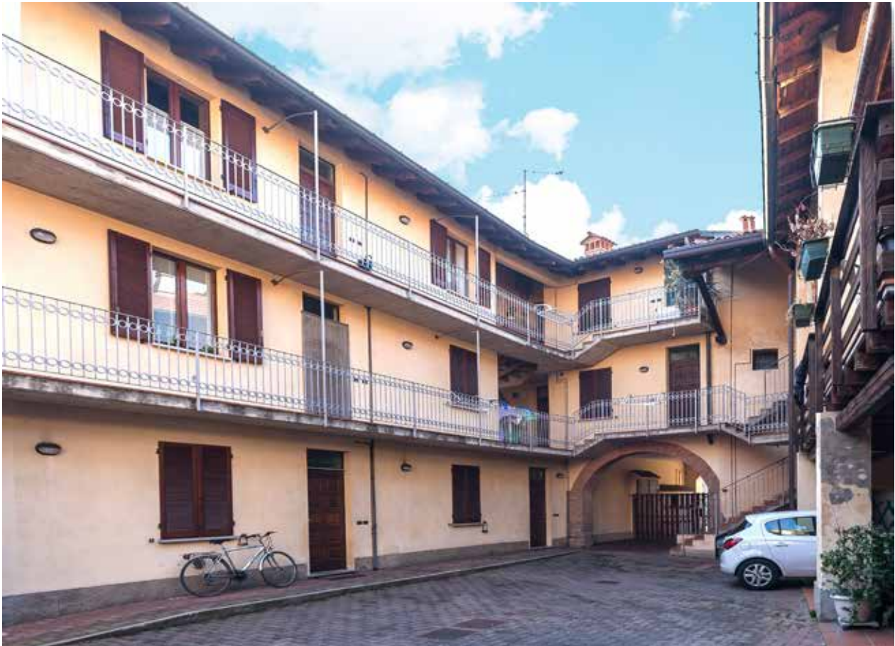
Condominio Briciola, Via Cavour 29
